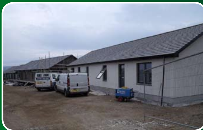
Shillinghill, Tobermory, on-site July 2011
