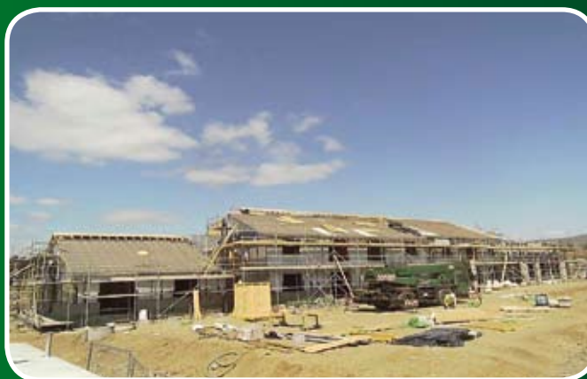
Mull & Iona Progressive Care Centre on-site July 2011
